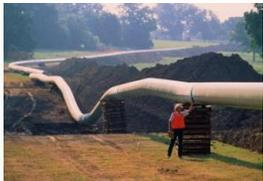
Keith Wood—Getty Images Worker checking welds on natural gas pipeline running through field
