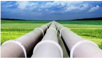
Sunoco Logistics Partners L.P. (NYSE: SXL) is about to put into operation Mariner East
